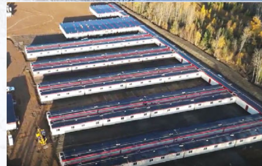
Construction camp assembly
