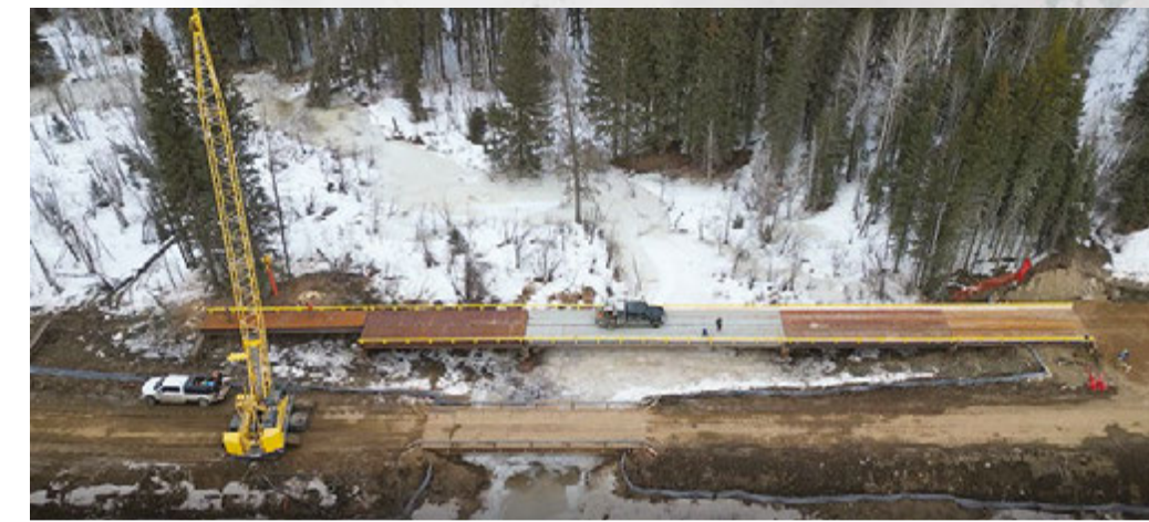
Blackrod - Road Construction
